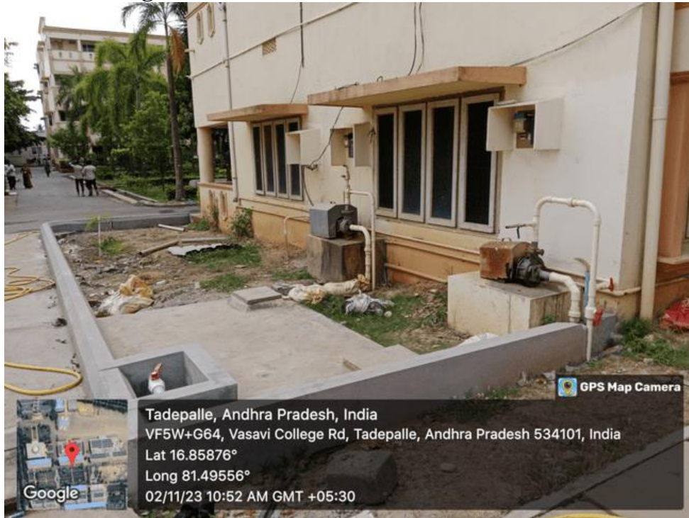
RO waste water to saved in tank for supplying water to washrooms and labs
